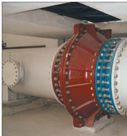
DN1400 (56") CLASAR® installation
